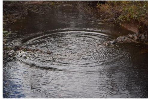
Figure 2: Member of the Blue Action Committee action committee (top left and top right) volunteered their time to construct a rock weir (bottom right) and minimizes the outflow drop at Culver 4 (bottom left).
