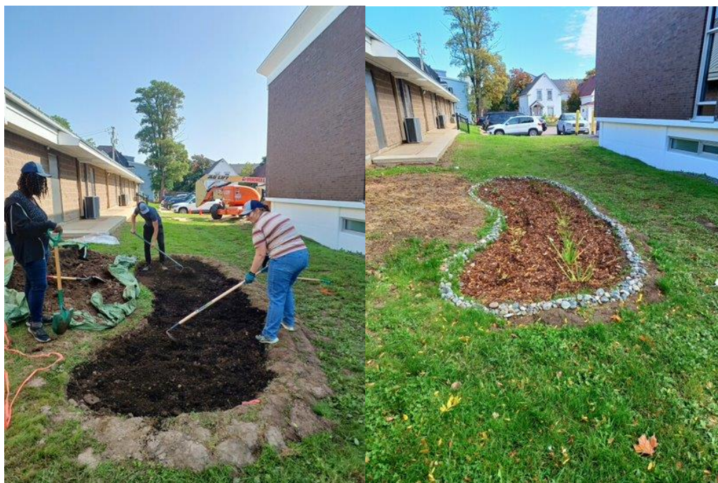
Figure 7: PWA staff and volunteers putting topsoil on the rain garden (left), completed rain garden on the Downtown Moncton (right)
