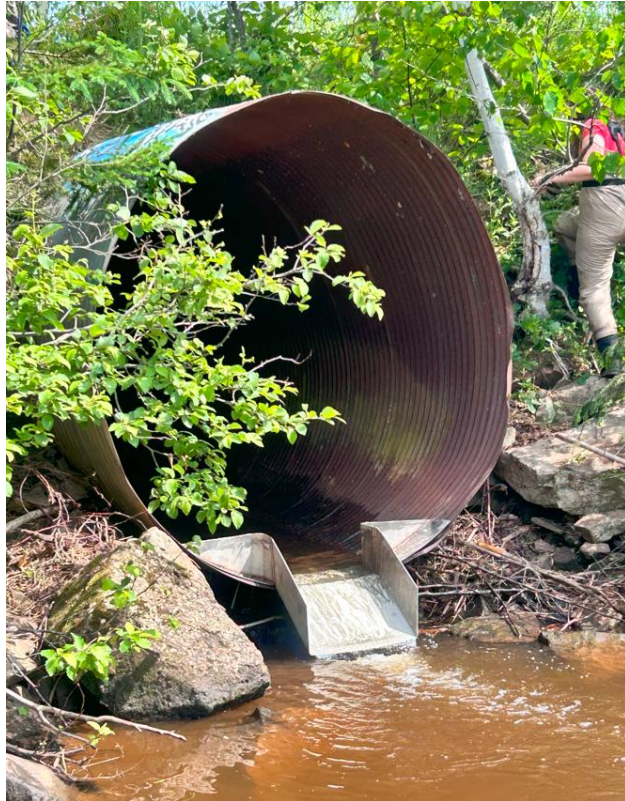
Figure 4: Outflow chute installed at a culvert.
