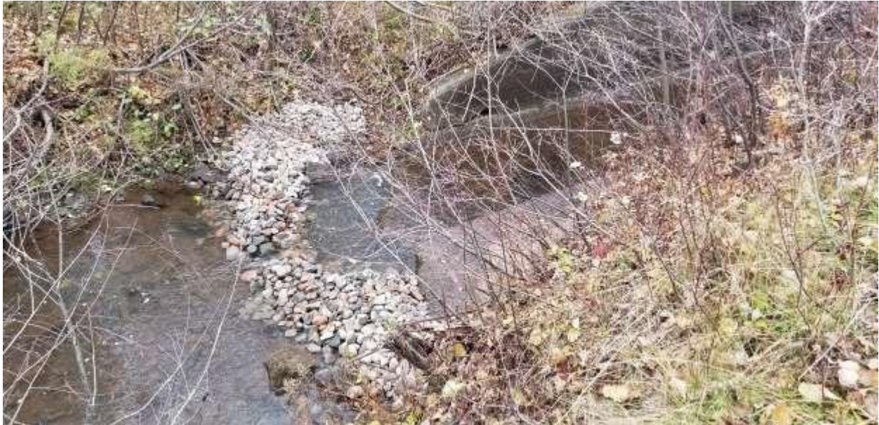
Figure 2: Rock weir constructed in 2020, located in the Halls Creek sub-watershed.
