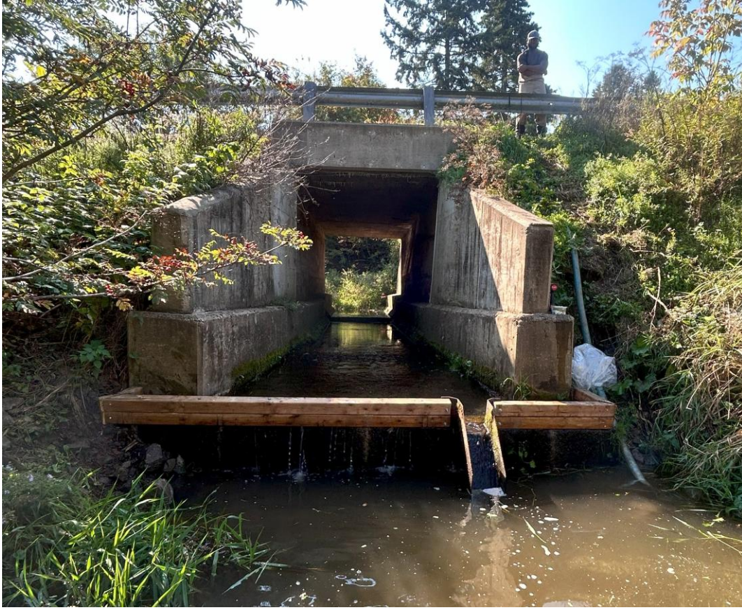
Figure 7: Outflow chute at culvert C-011 repaired in September 2024.
